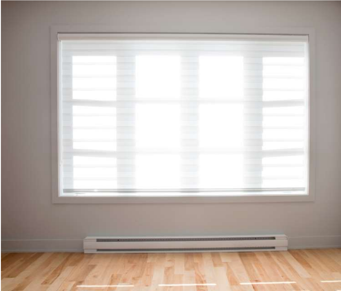
Figure 1 - Electric baseboard unit under widow
