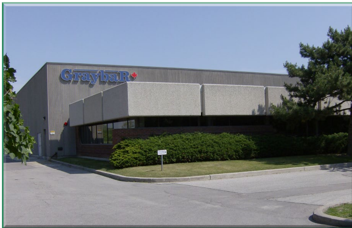
National Wire & Cable Warehouse 2750 John Street, Markham, Ontario L3R 2W4
