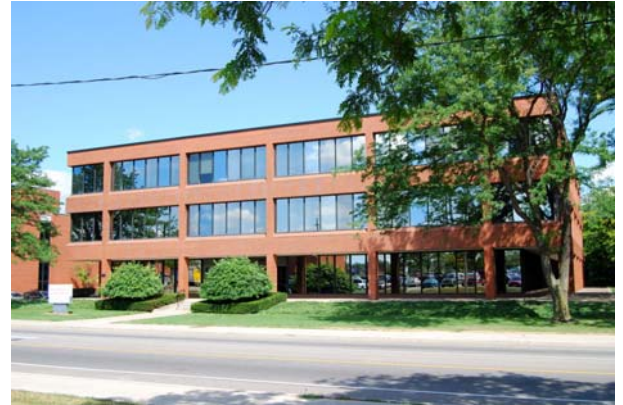
Hiram Walker Main Office - Windsor, ON
